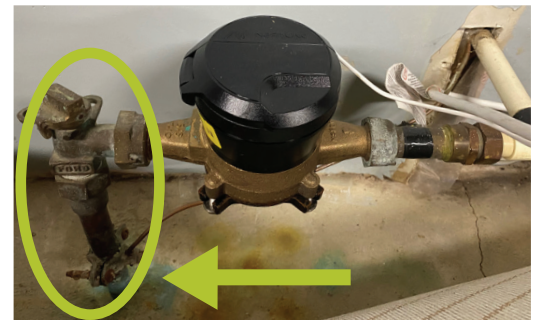
Service line here (copper) indicated by the arrow.
